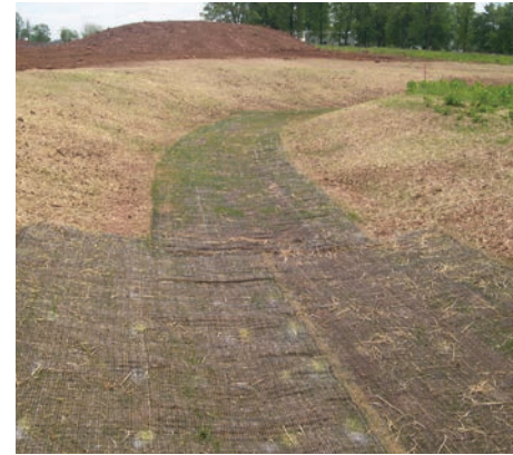
Correct Installation of Matting In a Swale ©LCCD, Rebecca Buchanan
